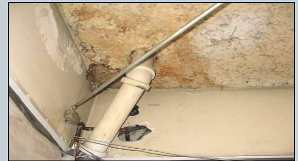
Water damage, deterioration
