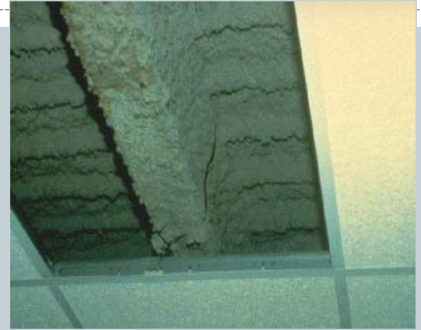
Sprayed-on fireproofing material
